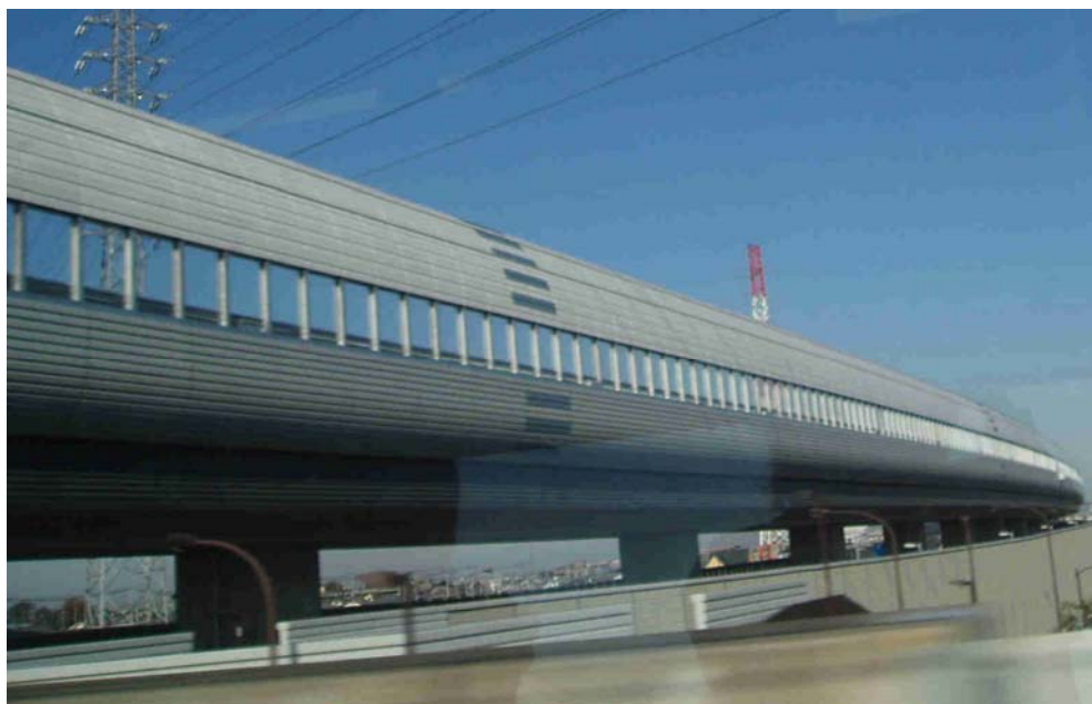
Figure 38. 30 km long new ring road in Tokyo area constructed with tall noise barriers bending over the road.
