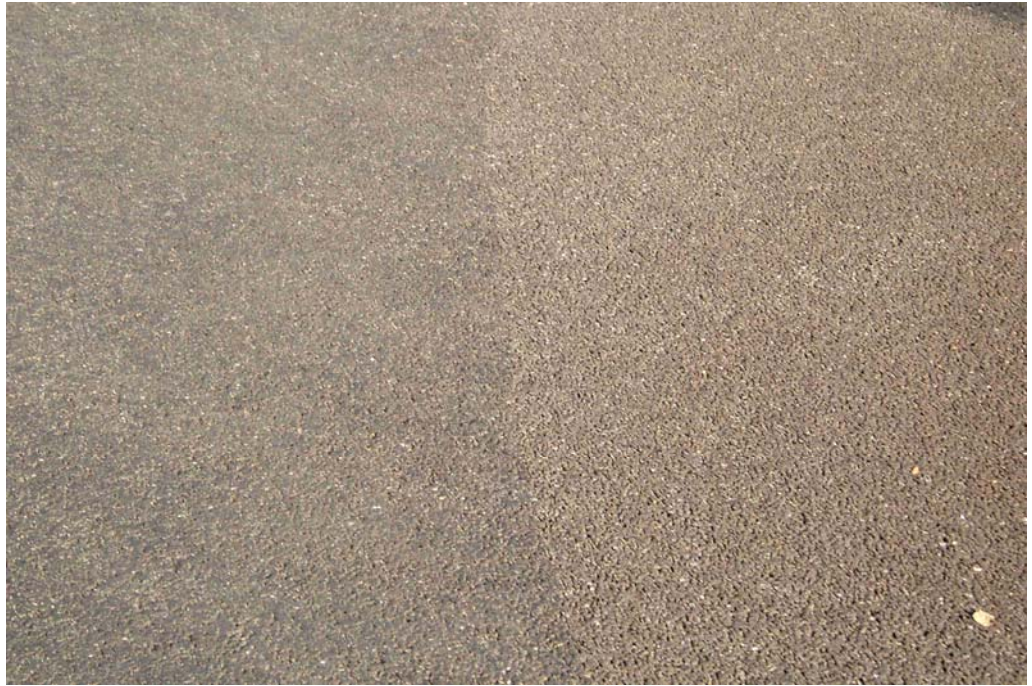
Figure 28. In an intersection part of the porous pavement was treated with the NIPPO product "Top Coat" in order to prevent ravelling caused by turning vehicles (left part of the pavement).
