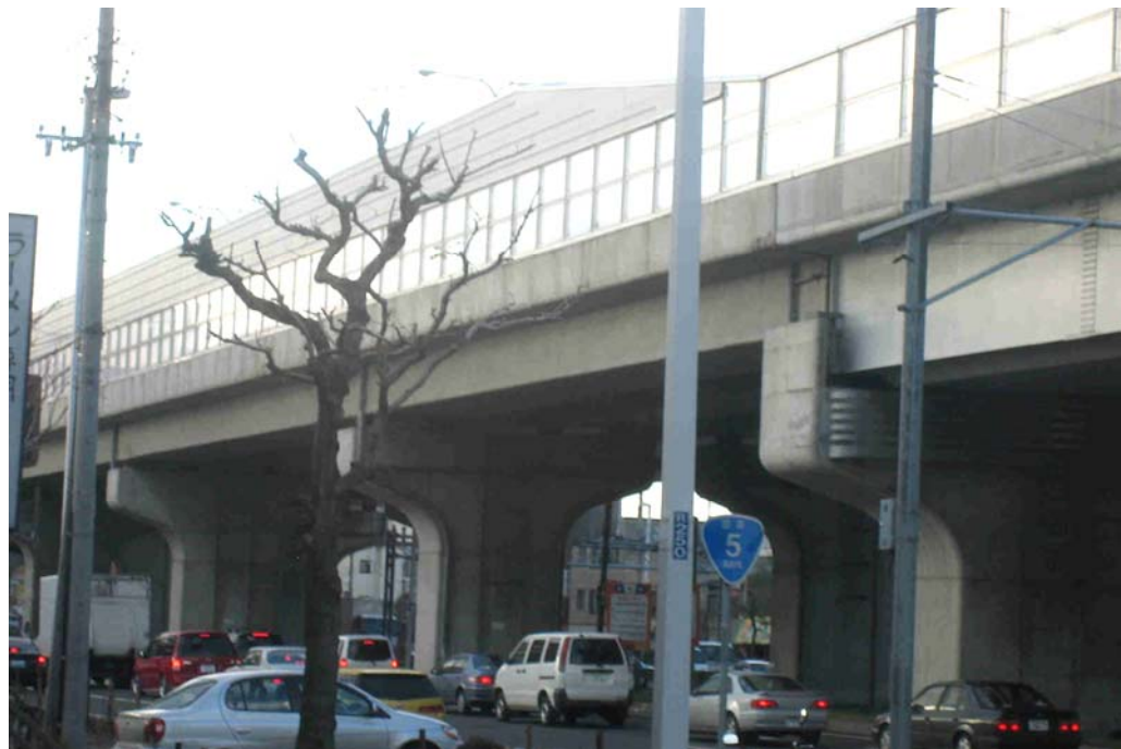
Figure 39. In the densely populated Tokyo area noise barriers are very common on the highway network.
