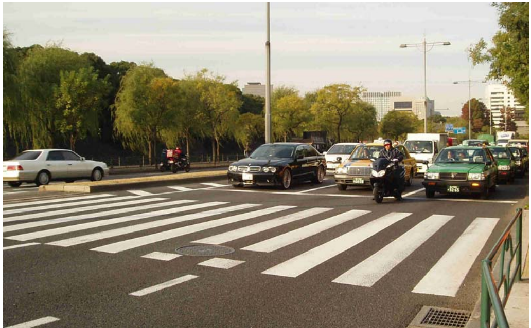
Figure 37. Porous pavement on a main road near the Emperors Palace in Tokyo with a driving speed of around 50 km/h. The porous pavement was also used at the adjacent intersections.
