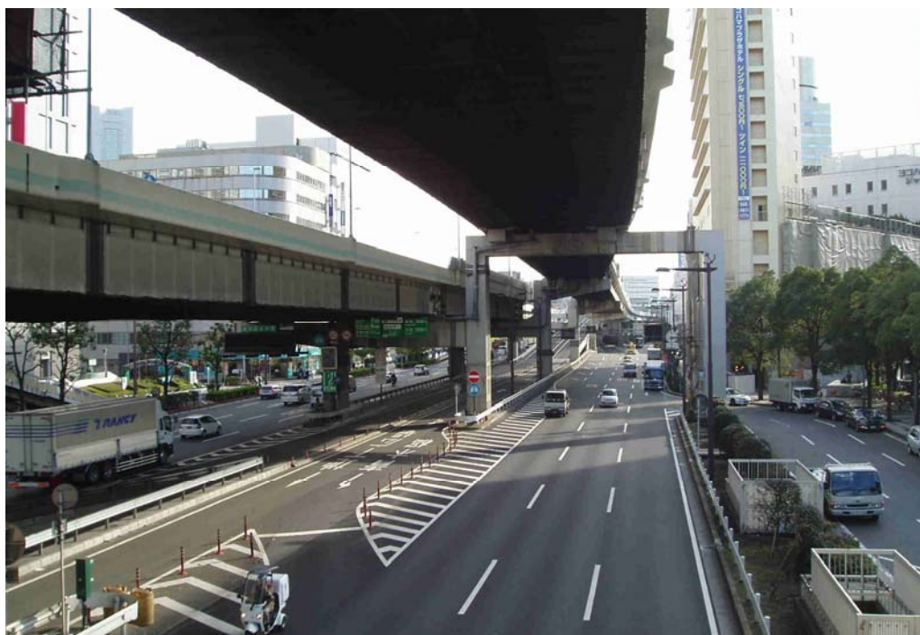
Figure 26. Highway with one year old two layer porous asphalt in Yokohama.
