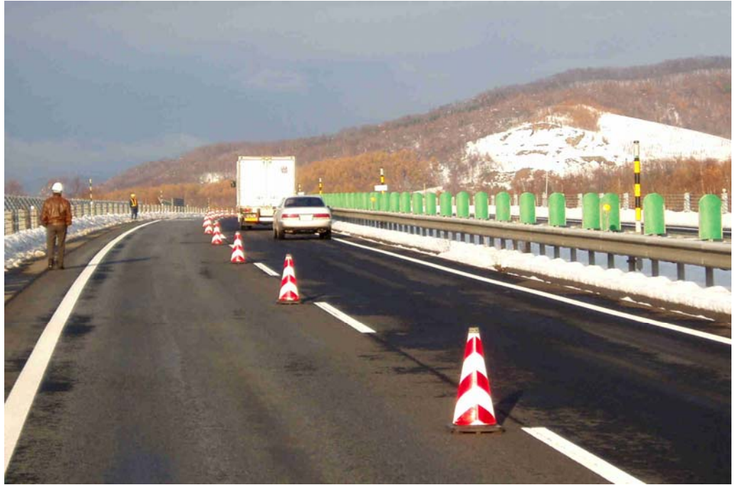
Figure 34. Highway 2 km north of Mikasa on Hokkaido Island with one year old porous and hybrid pavements with 13 mm maximum aggregate and a thickness of 50 mm.
