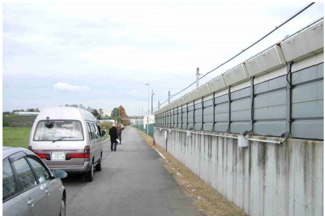
Figure 14. Noise barrier with active noise reduction device at the top. The 2.8 m high barrier is situated at the PWRI test track.
