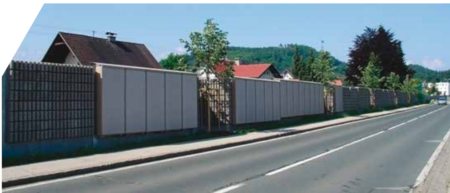
FIGURE 16. Test of a noise and dust absorbing barrier in Viktring, Austria. This study is part of the European project "Life-SPAS" [45]. © City of Klagenfurt, Dep. Environment Protection, Austria.
